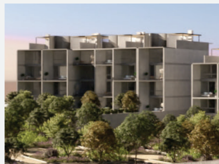
Depthouses Roof top ▲
